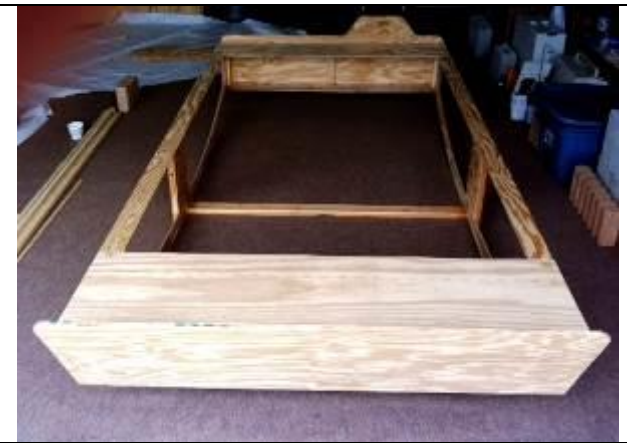
Stern transom view after side frames are attached. Note how the upper transom corners have been rounded off using a plastic cup to mark the radius.
